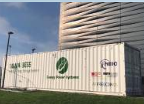
Exergy's 1MW battery energy storage system, installed at the E.ON Energy Research Center of RWTH Aachen University, Germany.
