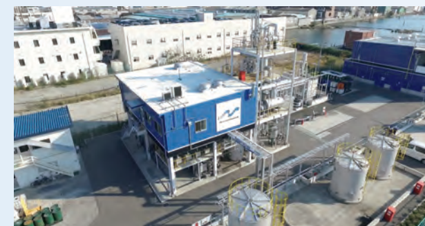
World's first commercial-scale microwave chemical plant(3200 t/yr)
