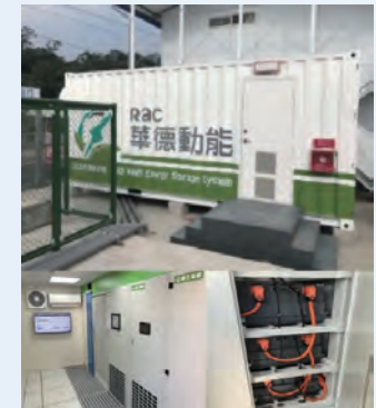
Case of Energy Storage (Utilization of E-bus battery)
